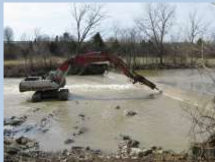
Olentangy River Dam Removal
