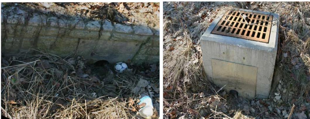
Figure 6. Unprotected Dry Basin Outlets
