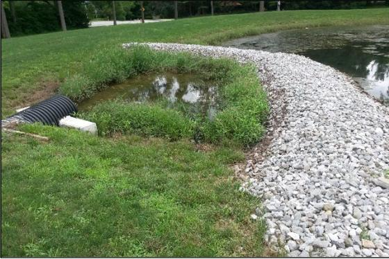
Image 2.6.1 Forebay with a rockfill berm.
