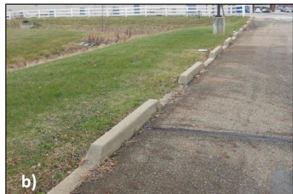
Figure 2.1.2 a) Raised Wheel Stop and b) Pavement Disconnected with Multiple Curb Cuts
