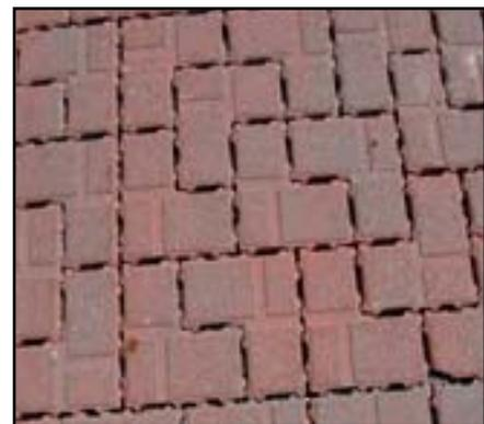
Figure 2.11.7 Pervious Interlocking Concrete Pavement
