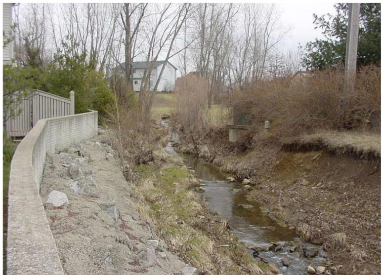
**Figure 1.1.1** This degrading stream is an obstacle rather than an amenity, requiring hardened banks and threatening utility infrastructure.
