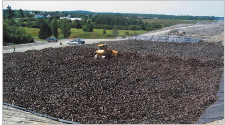
*Many beneficial products can be made from scrap tires, including civil engineering applications such as paving and drainage layers.*
