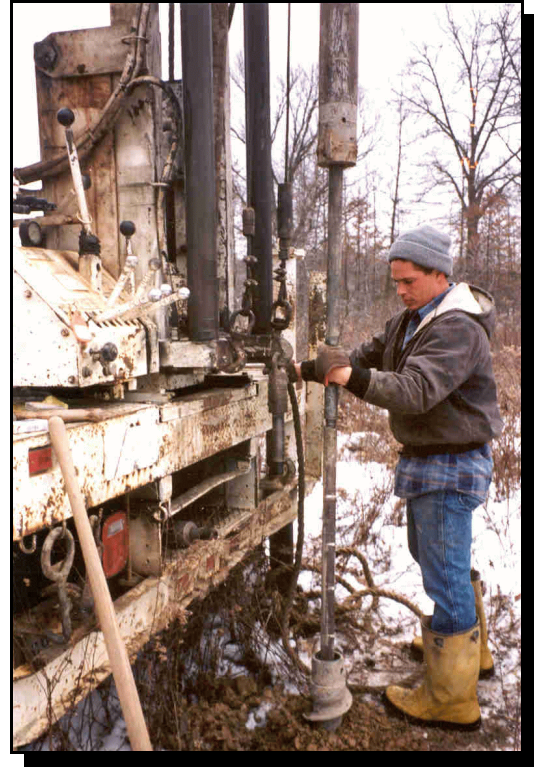
Figure 3-1 Drill rig and operator conducting a standard penetration test (SPT).
