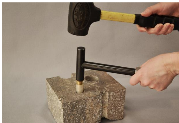
Figure 2. Installing the Vapor Pin™.
