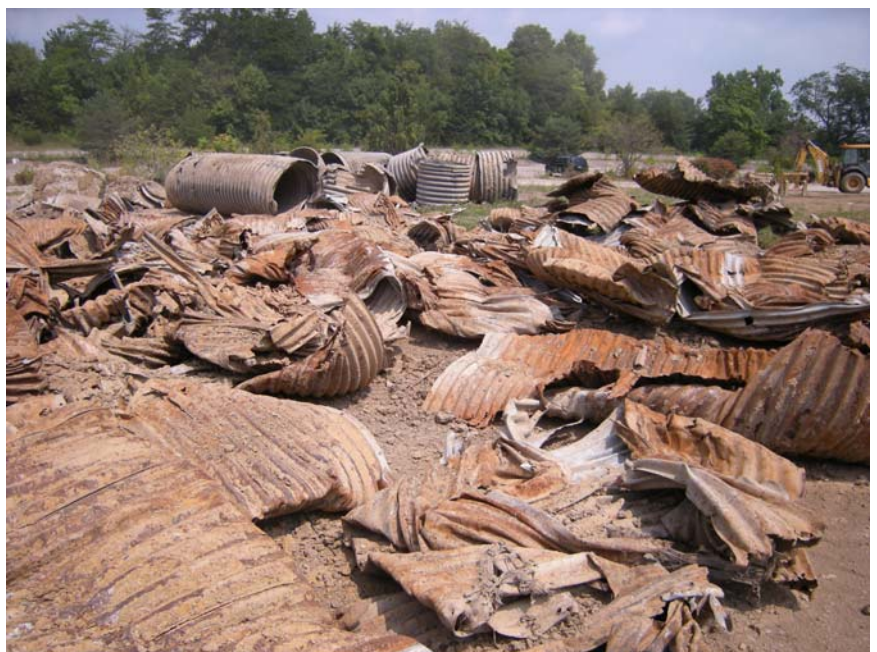
Culvert Pipe removed after day-lighting previously culverted stream.
