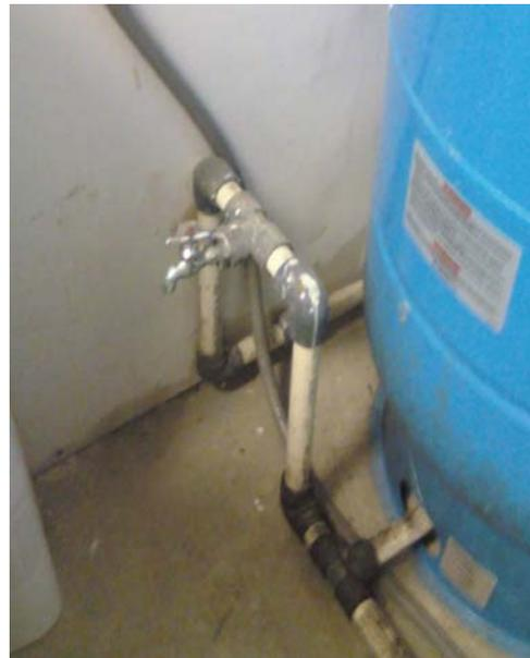
**Example #2:** The sample tap is constructed to have good clearance from the floor.
