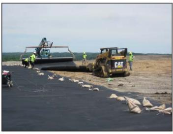
Flexible membrane liner (FML) being deployed at a landfill to control odors.
