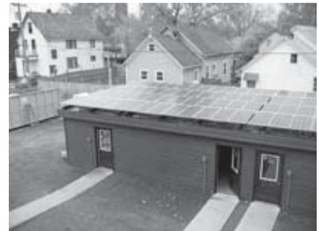
Photovoltaic arrays on the roof of detached town home garage.
